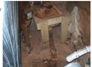
back room drain of dry cleaning business
